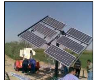
Iraqi crews deploy Solar Powered Water Purification units in Iraq
